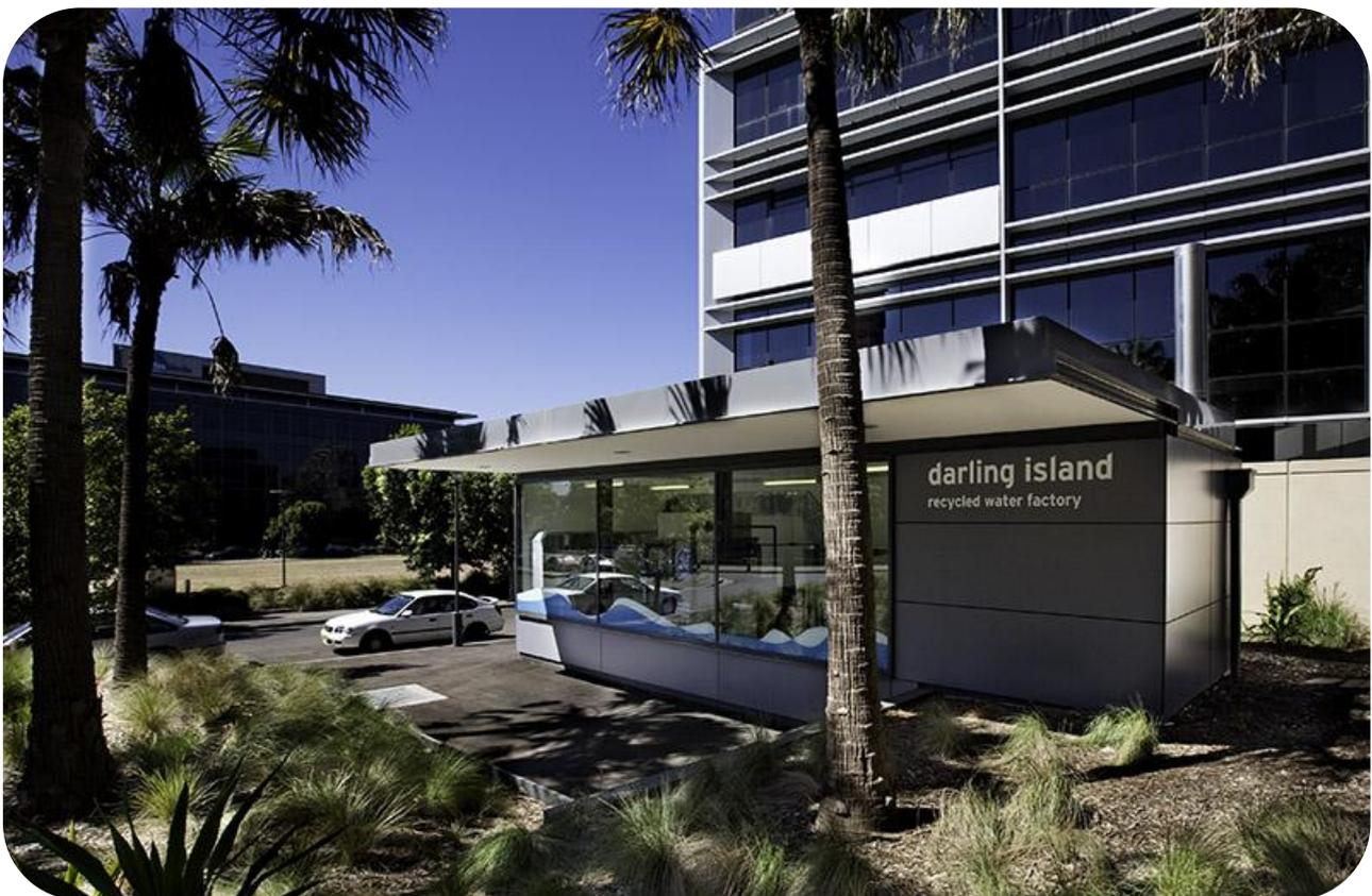
The on-site sewer mining facility at Workplace 6 produces over 10 million litres of recycled water each year
